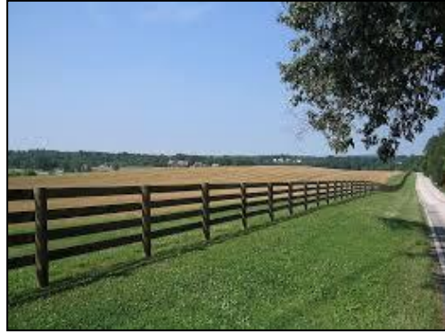
Figure 2: Four-rail fence; conforms to grade
