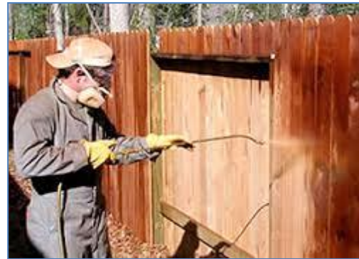
Figure 2: Painter staining fence; blotchy application
