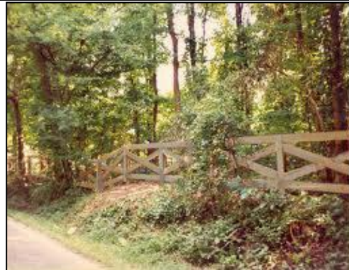
Figure 4: Cross buck, four-foot high fence; conforms to grade
