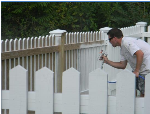
Figure 3: Spray painting open picket fence; as time consuming as staining
