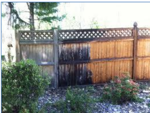
Figure 5: Example of how wood stains and deteriorates
